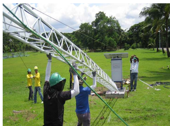
Installing Equipment _ AWS
