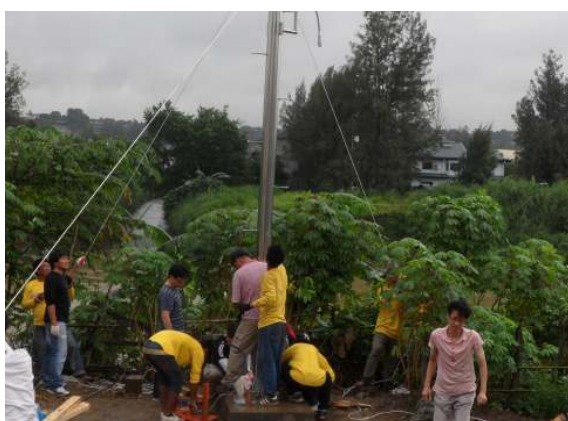
Installing Equipment _ Warning Post
